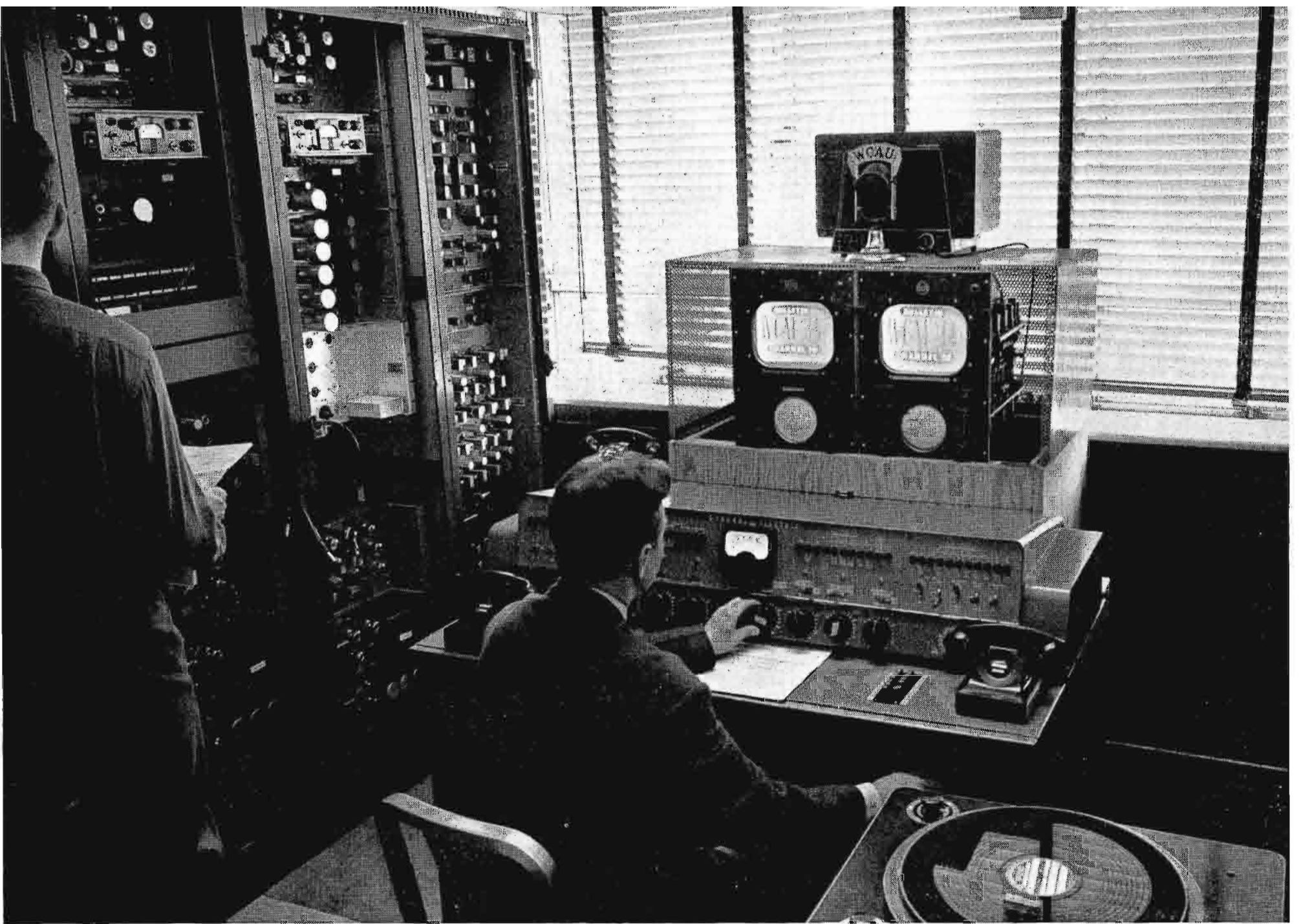
FIG. 28. View in the TV control room adjacent to the transmitter room. Operator sits at the desk containing video and audio monitoring and switching facilities. Terminal equipment and amplifiers occupy racks on either side.
