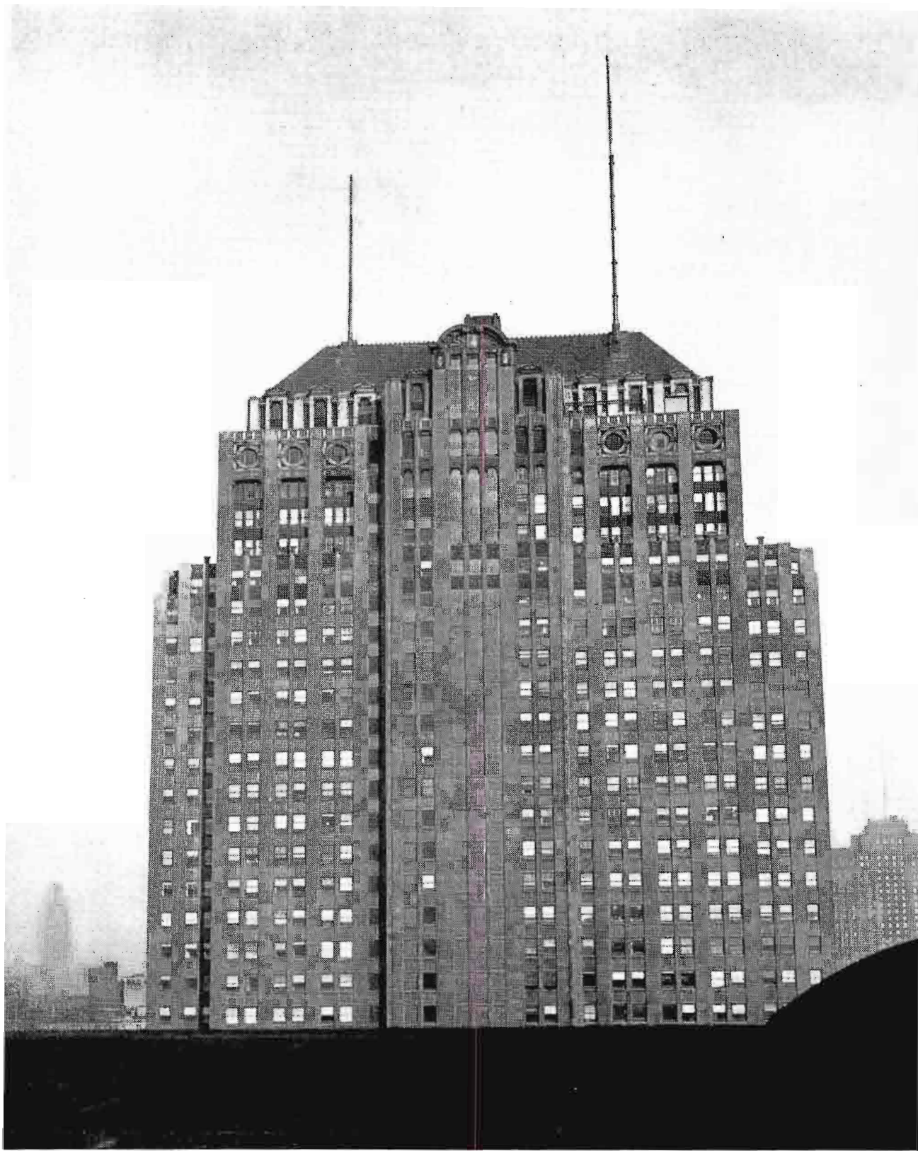
FIG. 3. The modern Opera Building at 20 North Wacker Drive where all of WENR-TV's facilities—studios, film rooms, transmitter room and antenna—are located. The 4-section Pylon with 6-section Superturnstile on top (right corner) of building is the combined antenna of WENR-FM and WENR-TV.
