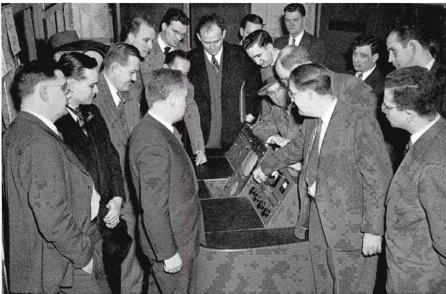
FIG. 3. In Building 53, where most of the RCA's AM, FM, and TV transmitters are assembled, the visitors participated in the tuning and operation of a 5 KW TT-5A television transmitter set up under typical operation conditions.
