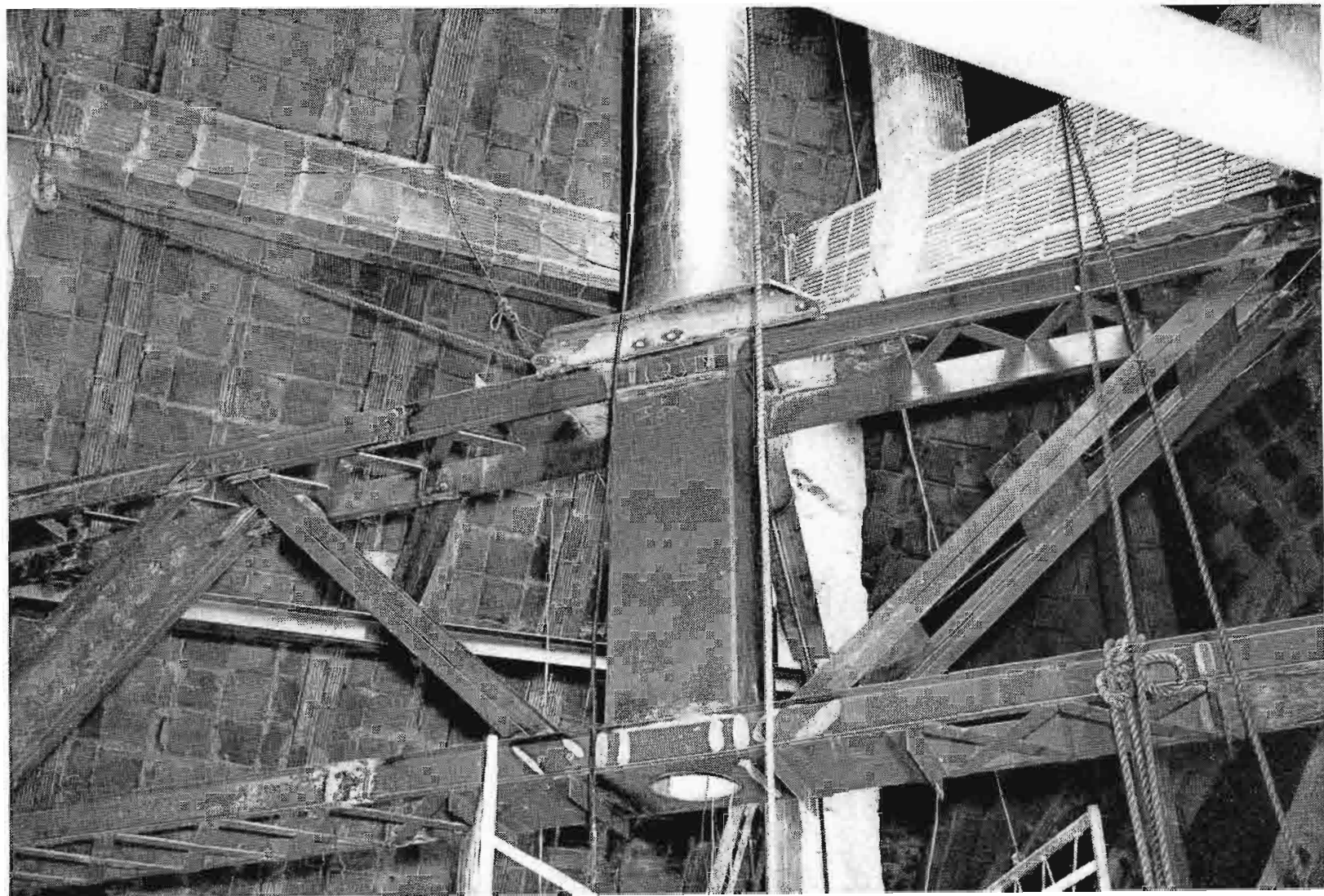
FIG. 26 (right). In order to secure the antenna supporting section onto the building the framework of the latter was reinforced and the welded steel frame shown here was mounted within.
