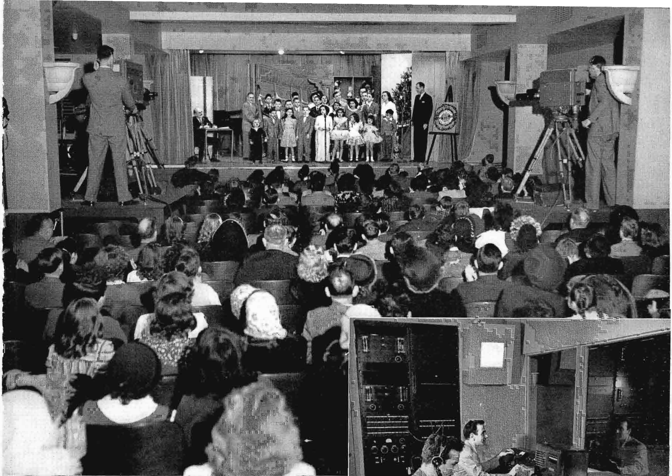
FIG. 10 (above). WCAU-TV's Studio X, shown above, is a 250-seat auditorium on the second floor of the building, designed originally for audience-type radio shows. It was easily modified for television and has worked out very well. Note cameras which are mounted on four-foot wooden platforms, two on the left of the auditorium and one on the right near the center.
