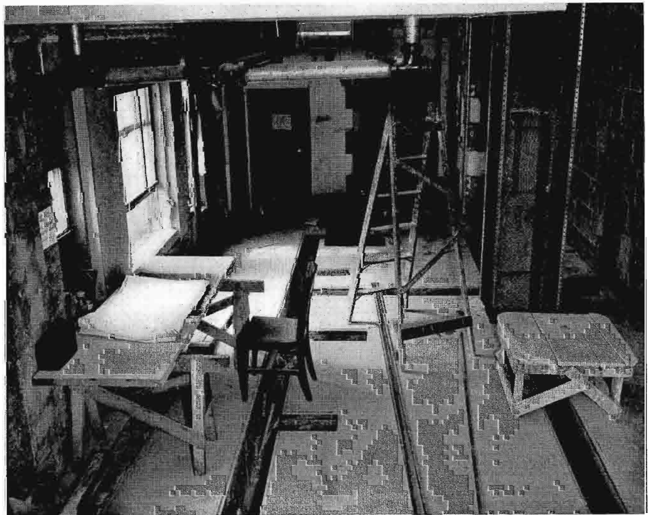
FIG. 7 (below). This is the film projection room during one stage of construction. Pouring of a false floor made it possible to provide wiring trenches and ducts between all main units. These trenches, shown open in this view, are provided with heavy steel coverings which protect wiring but are easily removable when changes or additions in wiring are required.
