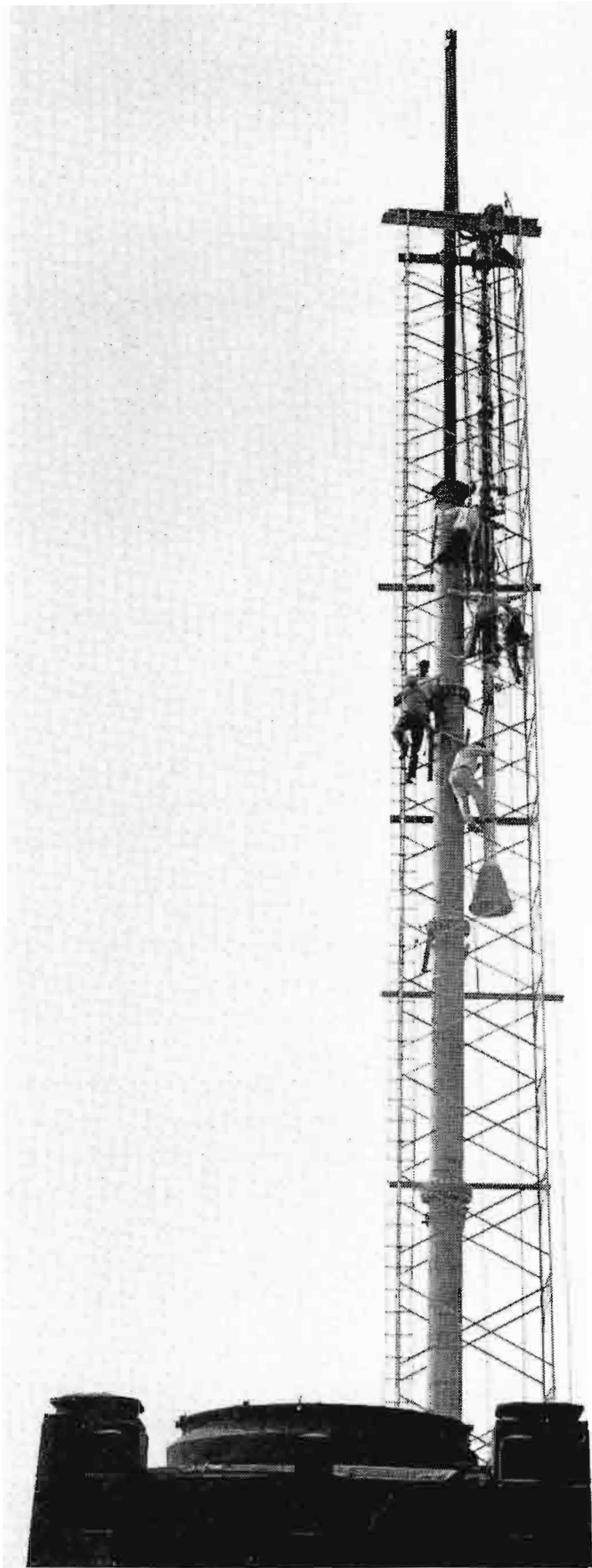
FIG. 24 (above). Erecting the antenna on the roof of the building was quite a problem. It was solved by building a tower-like scaffolding above a hole cut in the roof and bringing the sections up through the center of the scaffold.
