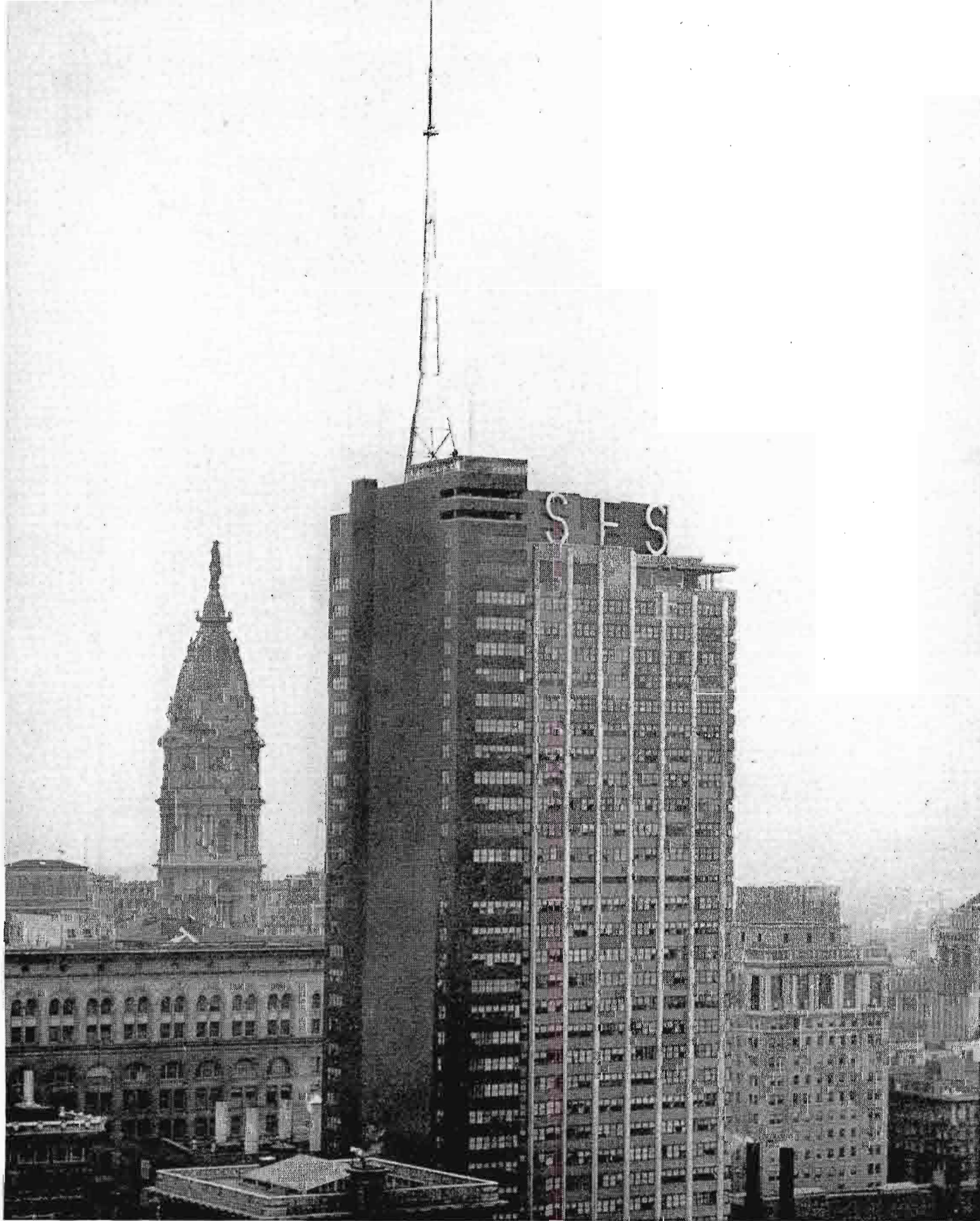
FIG. 23 (left). WCAU-TV's superturnstile antenna and WCAU-FM's two-section pylon antenna are mounted on top of a 181-ft. tower which surmounts the 479-ft. PSFS Building. Note famous statue of William Penn on City Hall in background.
