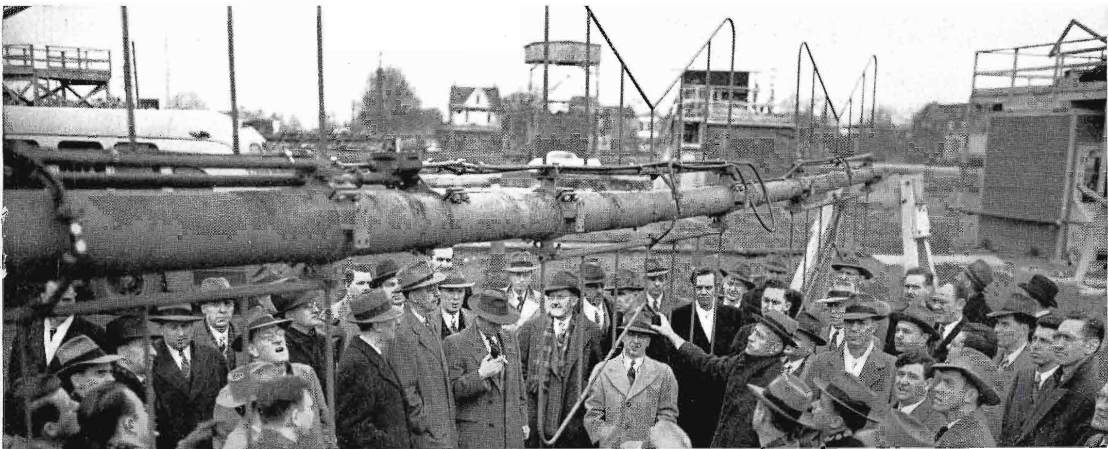
FIG. 2. While on tour of RCA manufacturing facilities, broadcasters got a closeup view of a Superturnstile television antenna being tested before shipment.
